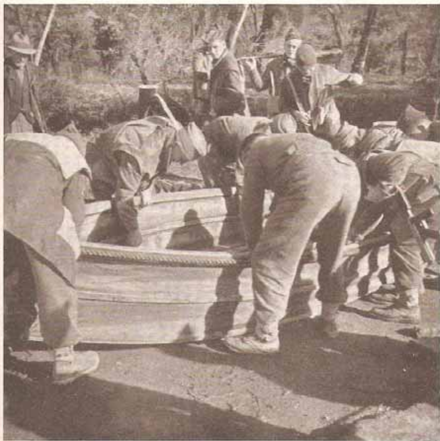
Erecting an assault boat
