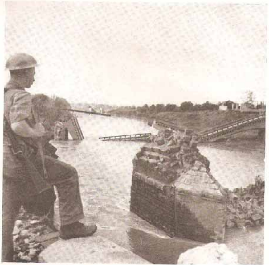
“Demolitions of characteristic thoroughness”
